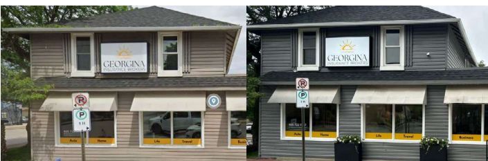
Before and after photos of CIP facade improvement in Jackson's Point
